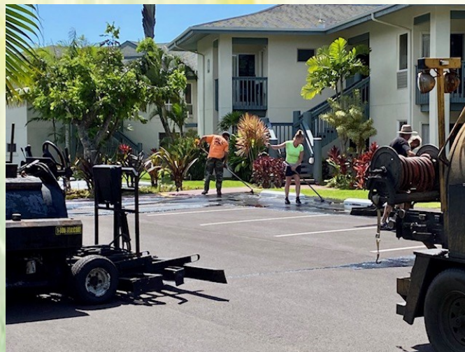
Paving/Striping of Exterior Parking Areas
